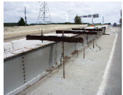
Strong-back beam support on bridge deck
