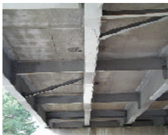
View of Beam AFTER Repair
